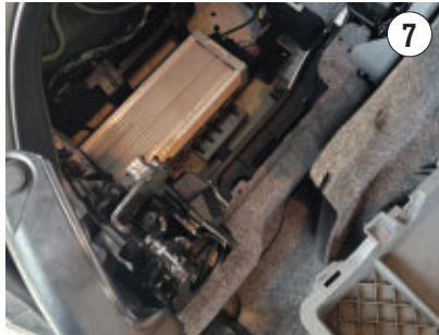
7 THIS AUDIO SYSTEM amplifier is located in the trunk and was accessed for circuit testing.
