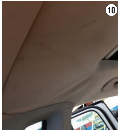
THESE WATER STAINS on the headliner are a telltale sign of a water leak.
