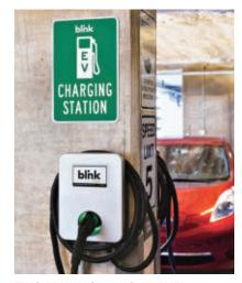
**THIS BLINK IQ 200 IS A LEVEL 2** charger that can be installed on a wall or pedestal mount. A 240-volt connection is required to power the charger.
