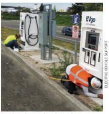
**ELECTRIC VEHICLE SUPPORT** is installing Level 3 charging stations in the state of Washington. They are a general electrical and construction contractor that specializes in the design, permitting, installation, and service of vehicle charging stations of all types.
