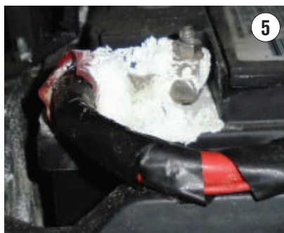
DO NOT RECOMMEND A BATTERY SERVICE when you see this. A new cable and possibly a battery replacement are needed to fix this one.
