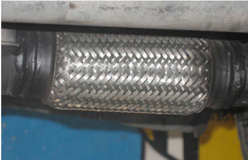
Common sources of air leaks into the exhaust system that can skew the ECM's tests include damaged flex pipes and stripped or damaged sensor threads.
